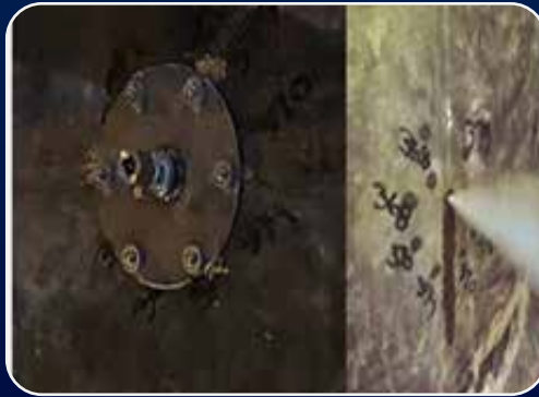
Online repair of pressure equipment
