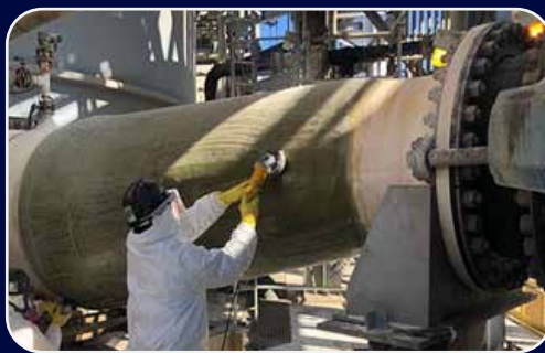
FRP Piping repair jobs
