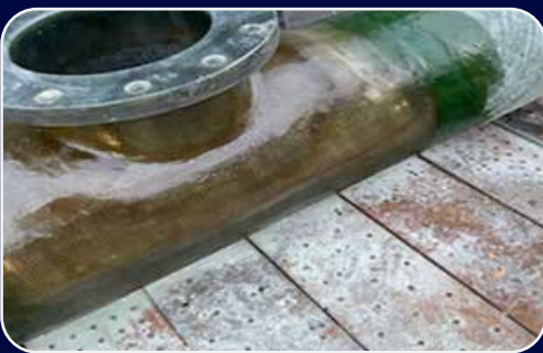
FRP Piping repair jobs
