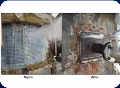
Online repair of pressure equipment
