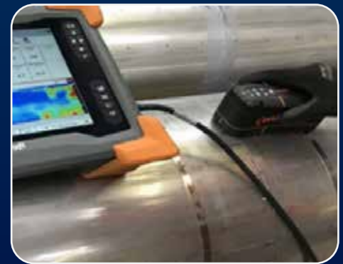
Providing advanced technique to inspect corrosion under insulation.
