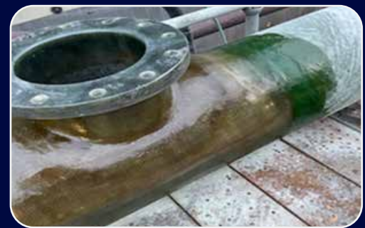
FRP Piping repair jobs
